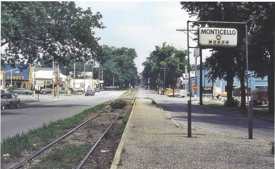
Right: The plastic-and-aluminum illuminated, two-pole station platform sign remained intact until destroyed in a 1974 tornado. This view looks north on Railroad Street. — John Fuller photo
